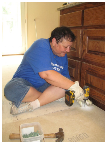
Sandy (aka "Rosie the Riverter") laying down cement board in preparation for ceramic tile ->
