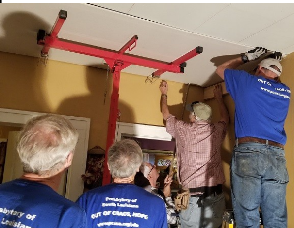
Part of the team worked at dry-walling the ceilings in most of the rooms.
