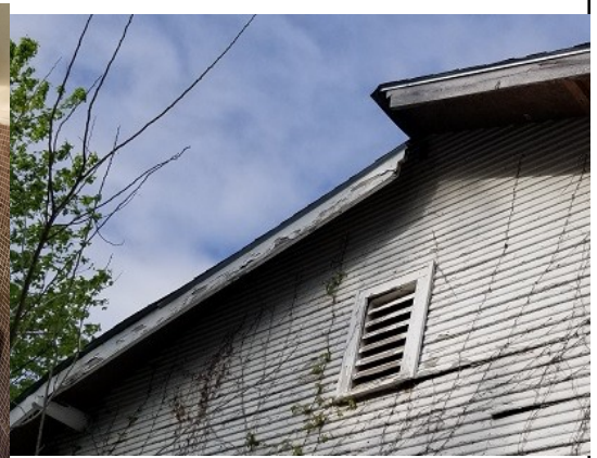
This was the biggest problem with Jackie house. A broken soffit and leaking roof.
