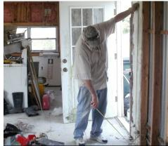
Allen frames the doorway. The old trailer door had been broken in by thieves. We replaced it with a steel, house-quality, front door.
